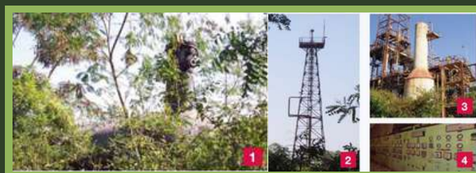
Figure 2: 1. MIC Storage Tank 2. Location of MIC Release 3. Sodium Hydroxide Scrubber (not functioning at the time of the incident) 4. View of the Control Room [4]
